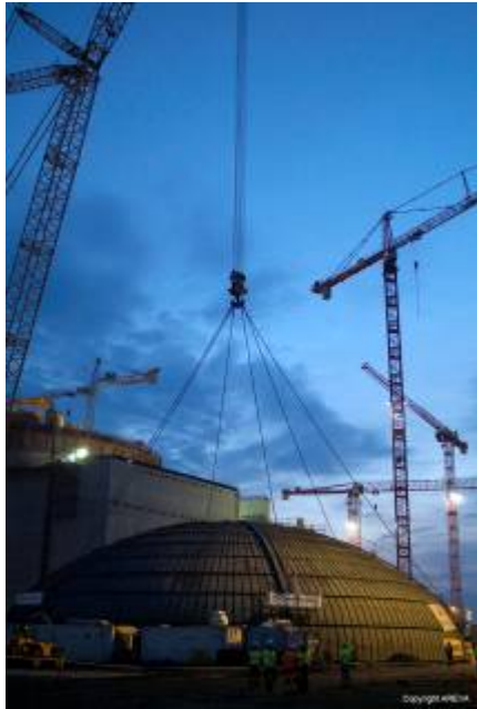
Inner Dome Installation
