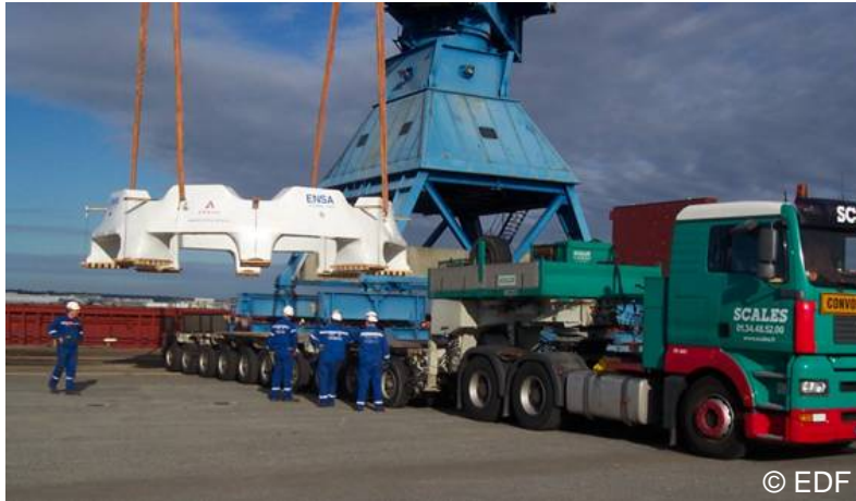
Reactor Pressure Vessel Support Ring delivery
