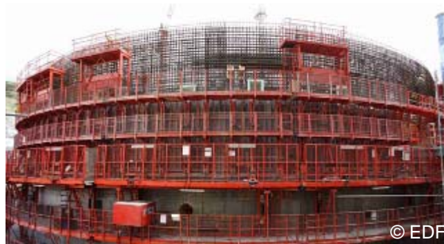
TOP: General view, East West RIGHT: Reactor building foreground, turbine hall background BOTTOM: Reactor building external form works AUGUST 2009
