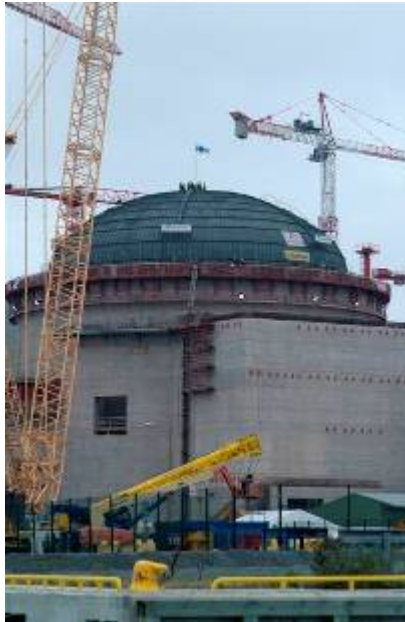
Inner Dome Installation
